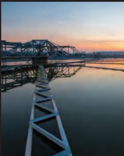
ABU DHABI Water Supply Project
