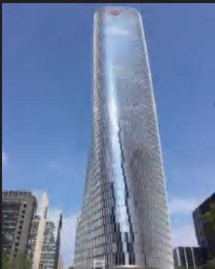
Bank of China Data Center
