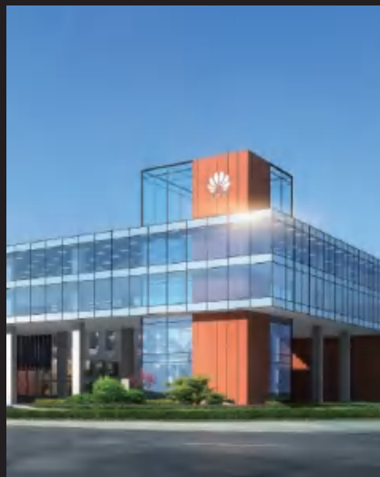
Huawei Cloud Computing Center
